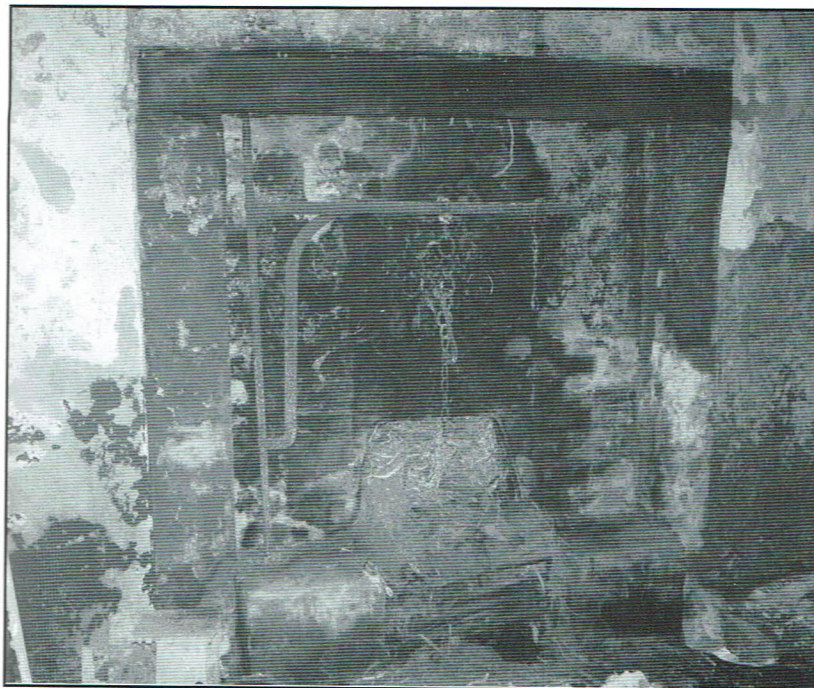
The fireplace was fairly typical of the time. The crane has still two sets of chains and one crook attached. Two hobs are also shown; these were useful to set pots and pans on to keep food warm. The surround has been removed.
